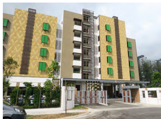
The nearly completed SANH (Taman Jurong). Photo taken in November 2018.
