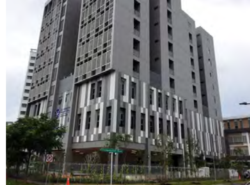
Construction of SAAH (Sengkang) is on schedule and the home is expected to be operational by April 2019.
